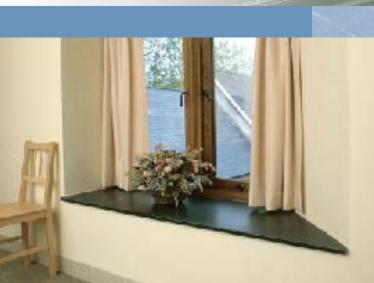
A further advantage is the option slate sills offer the builder for closing the wall cavity. This has become increasingly important with the building regulations regarding closed cavities around windows and prevention of moisture absorption.
